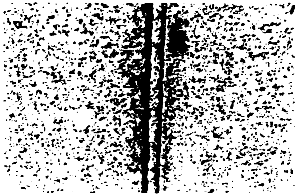
Fig. 3.2.3.3 — Joint sealant bond loss
